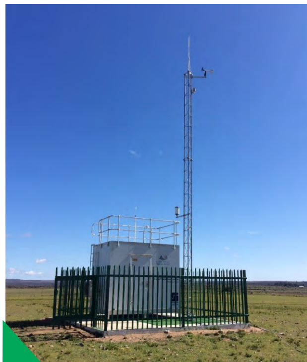
An Air Quality monitoring station
