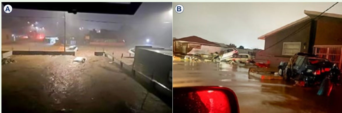
Photo 1 A and B: Torrential rain severely damaged Uitenhage in the Eastern Cape on Saturday night, 1 June 2024. (Source: Smile FM, Daily Maverick, 2024)
