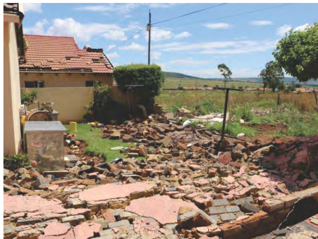
Ennerdale tornado damage
