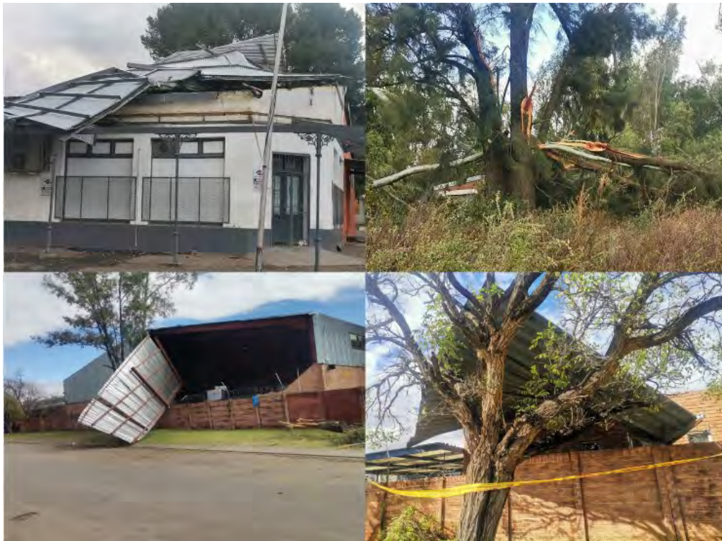
Figure 8: Ground evidence in Hilton and East-End (Michael & Rejoyce)
